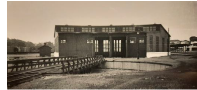
Joplin Union Depot is in the background on the right.
